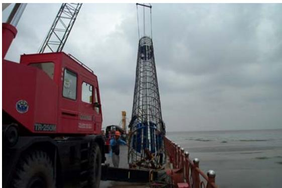
**Figure 2** Multi-level bi-directional test over water.
