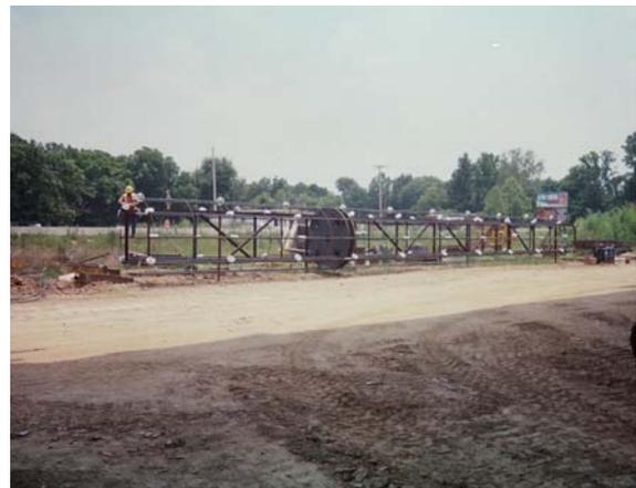
**Figure 17** Dedicated carrying frame and O-cell assembly ready for installation
