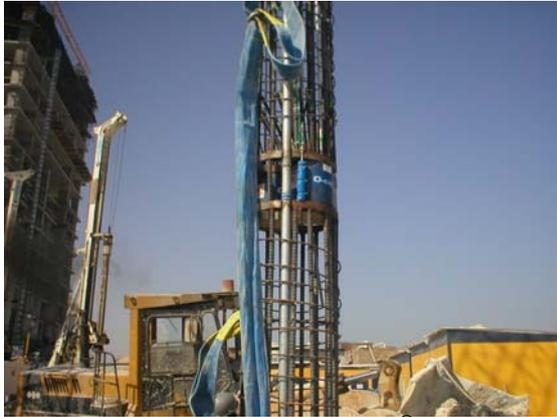
**Figure 4.** Cage showing O-cell<sup>®</sup> assembly attached for a 0.9m pile – State of Qatar
