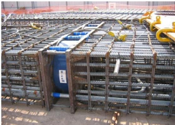
**Figure 15** Placement of O-cells in a barrette cage, test capacity 88 MN – Dubai, UAE
