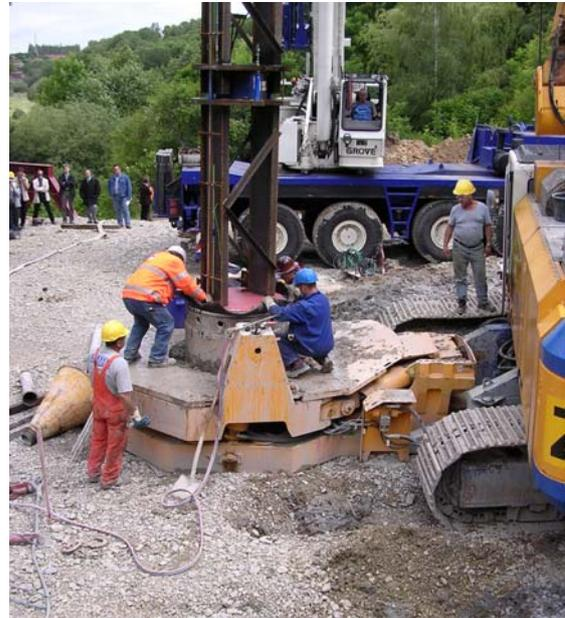
**Figure 16** Carrying Frame used at Weida Bridge, Germany for a multi-level bi-directional test.
