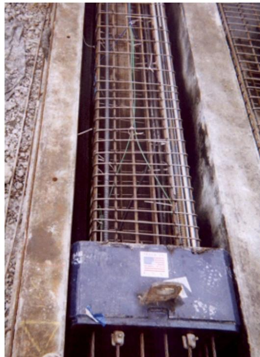
**Figure 13** Placement of O-cell<sup>®</sup> in pre-cast pile at manufacture
